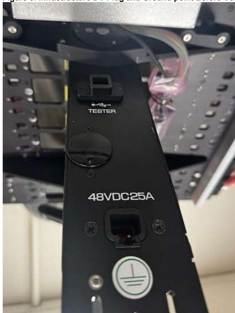
Figure 6: Infrastructure DC Plug and Ground point Before Connecting
